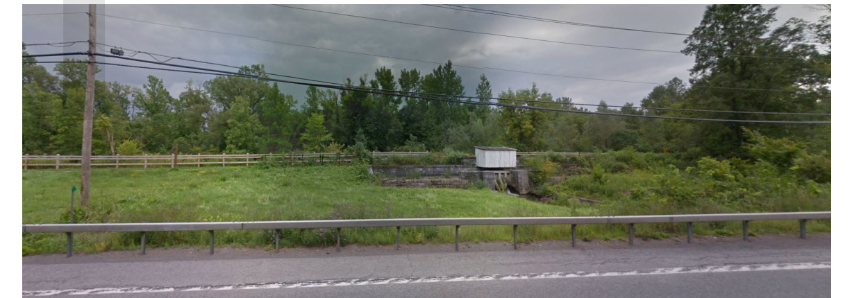
Mud Creek Aqueduct
